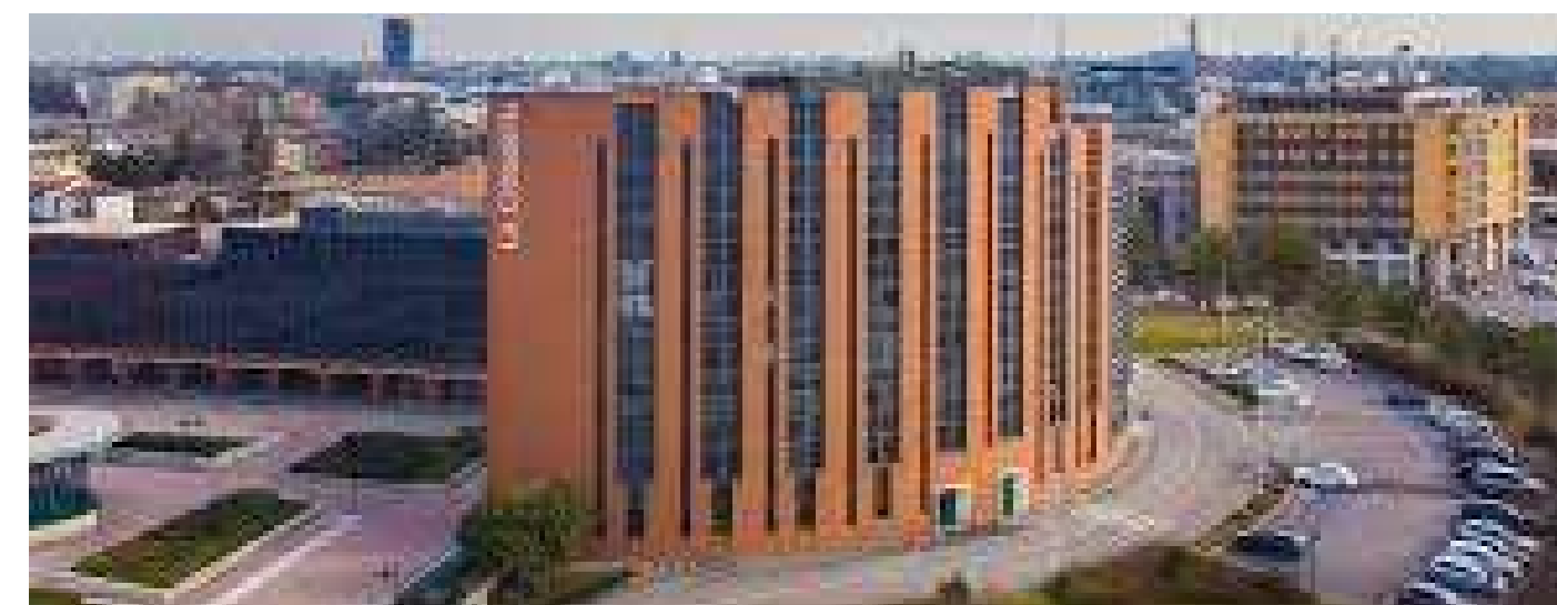
Fòrema headquarter in the heart of the « Innovation Boulevard » in Padua – Veneto Region
